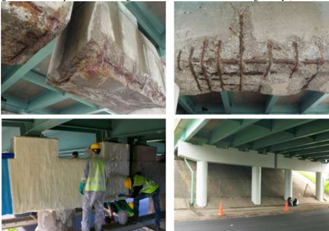
Figure 10. Rehabilitation using FRP wraps of Madison Avenue Bridge, Huntington, WV (WVU, 2014)
