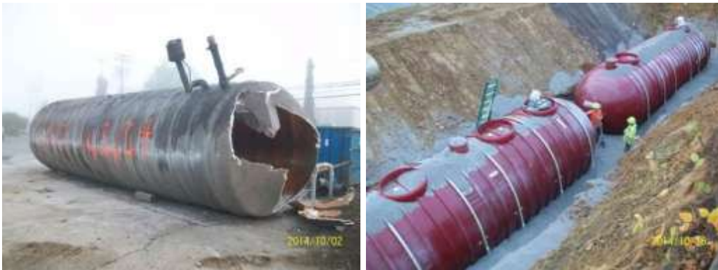
Figure 6. Durable FRP Gas Tanks (Liang, 2014)
