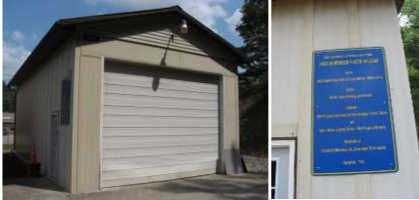
Figure 8. Multi-purpose FRP building with modular panels, Weston, WV (WVU, 1995)
