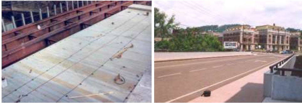
Figure 1. Market Street Bridge (Wheeling, WV, built in 2000) with FRP decks (WVU)
