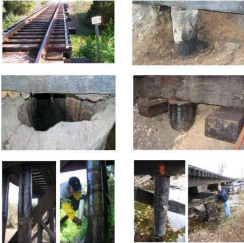
Figure 11. Retrofitting of railroad bridges using FRP wraps, Moorefield, WV (WVU, 2010)
