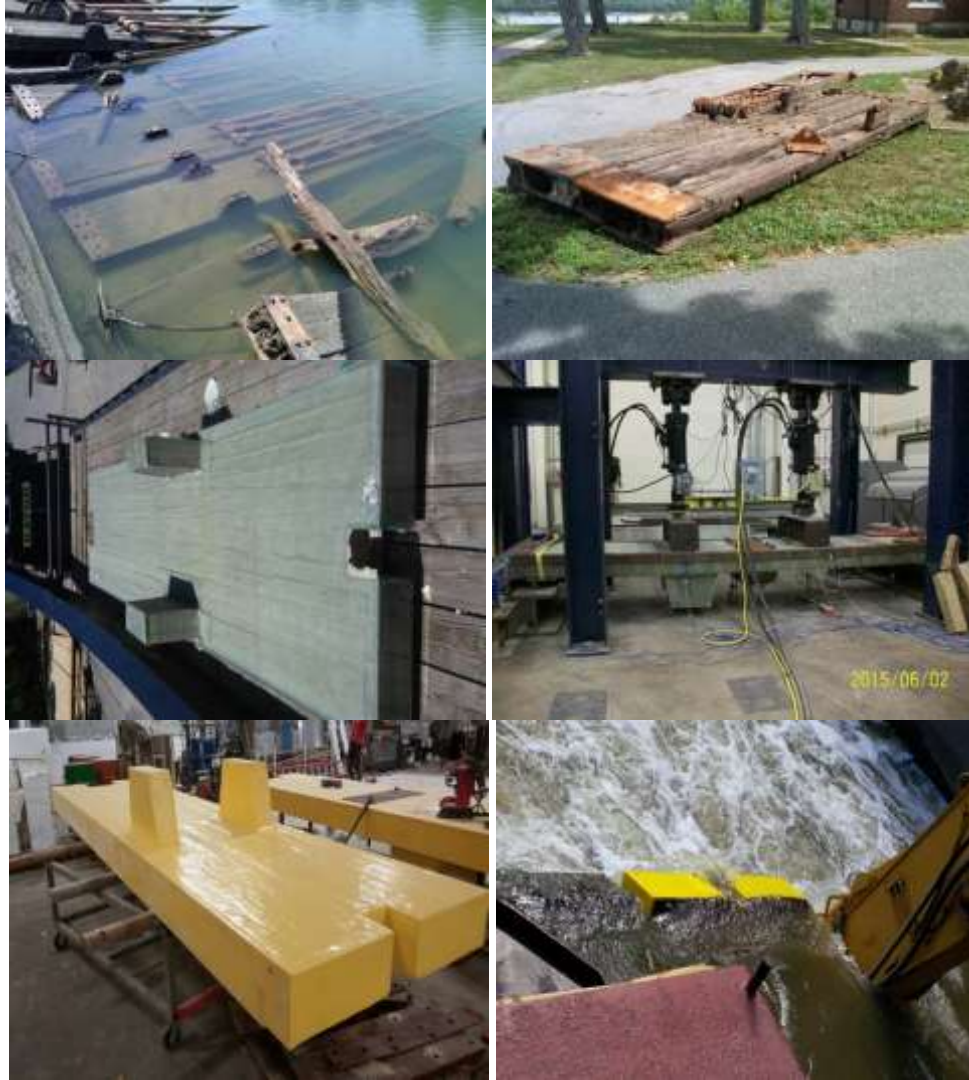
Figure 13. Composite Wicket gates and its field implementation in lieu of deteriorated wood wicket gate. The composite gate is \frac{1}{2} the cost with a much longer expected design life. (WVU, 2015)
