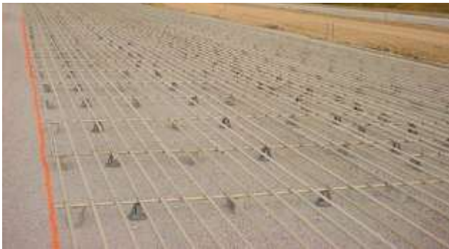
Fig 2. Pavement with FRP Rebar, WV Route 9, Martinsburg, WV (WVU, 2007)
