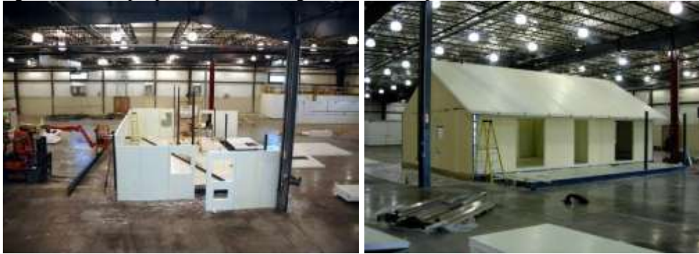
Figure 9. FRP composite house being erected at BRP Inc. manufacturing facility (WVU, 2008)
