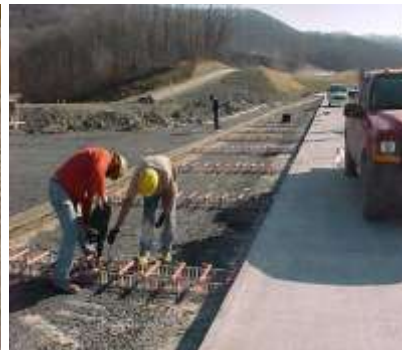
Fig 3. Pavement with FRP Dowels Elkins Corridor H-Project, Elkins, WV (WVU, 2003)
